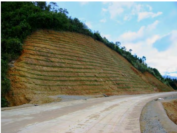
But these massive and costly retaining walls by themselves did not stop erosion during the typhoon season
