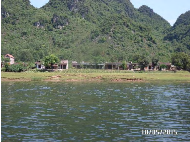
Erosion along unprotected river banks
