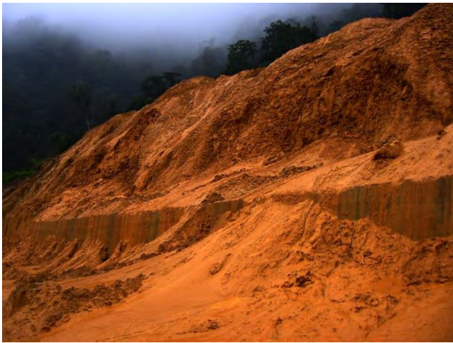
But these massive and costly retaining walls by themselves did not stop erosion during the typhoon season
