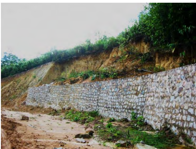
Conventional hard structure solution: Small and large retaining walls
