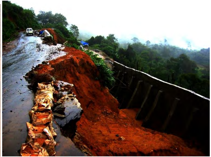
But these massive and costly retaining walls by themselves did not stop erosion during the typhoon season
